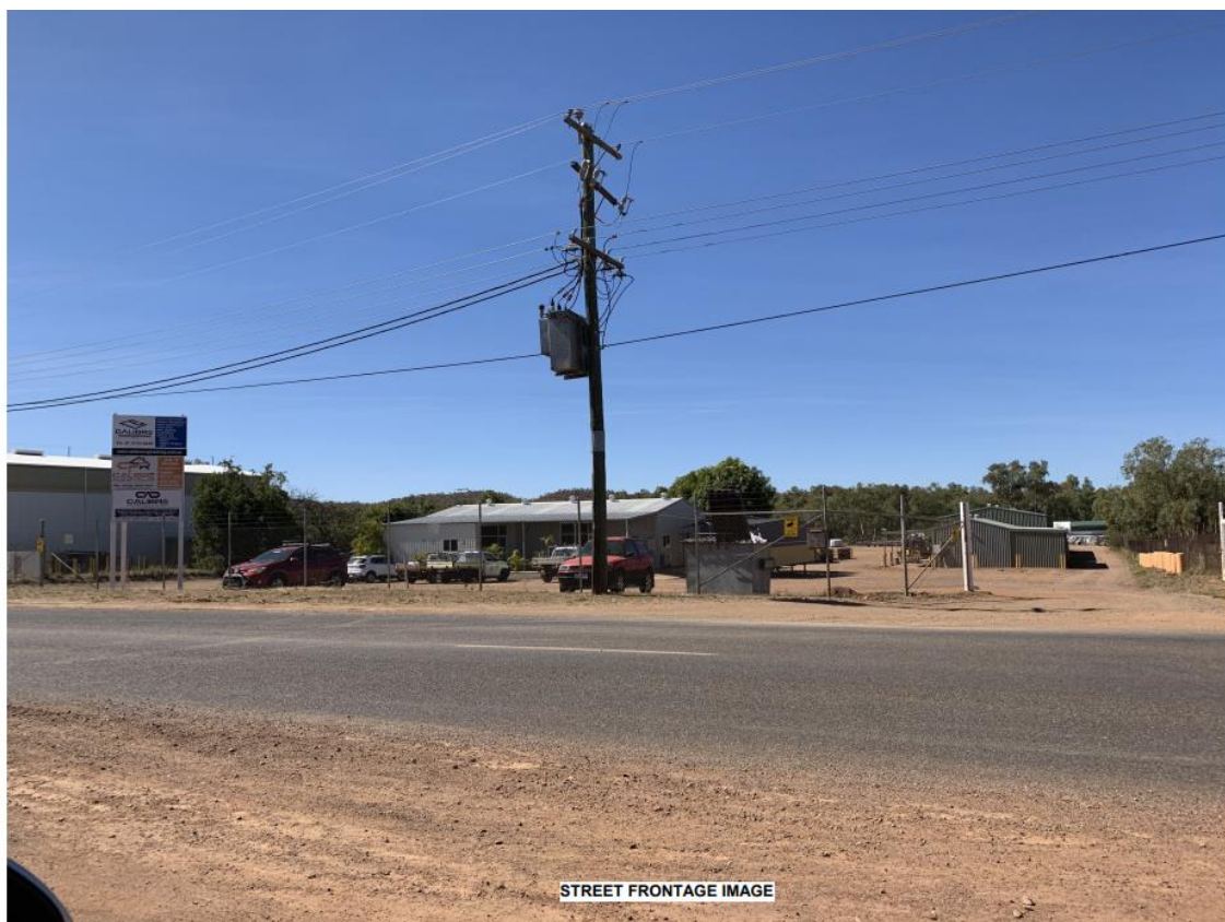
FIGURE 3 – EXISTING ENTRANCE OFF OLD MICA CREEK ROAD
