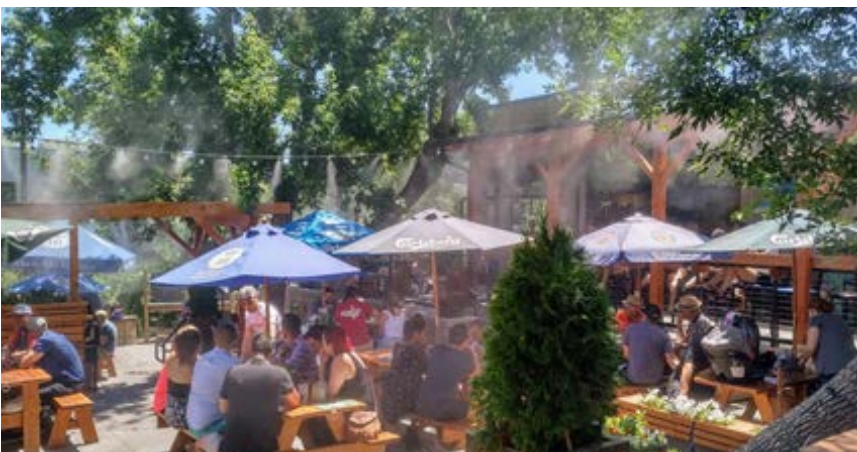
Image 2. Commercial installation of misting cooling system
