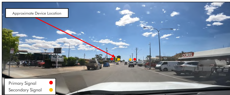
Figure 3.4: ADVANCE VISIBILITY ON NORTHBOUND APPROACH
