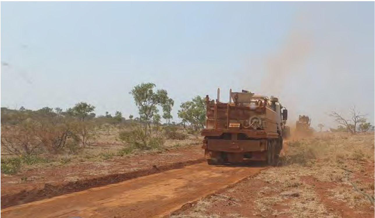
Figure 5 - Creating Firebreak on Lagoon Creek Station
