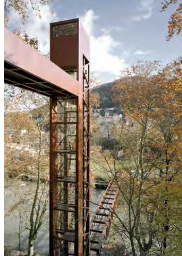
Gironella old town centre, Spain https://www.publicspace.org/works/-/project/249-new-lift-to-the-old-city-centre https://www.archdaily.com/776902/new-access-to-gironellas-historic-center
