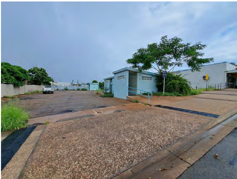
Figure 2- Site Photo showing poor state of existing toilet block, substation and carpark at 34 Miles Street
