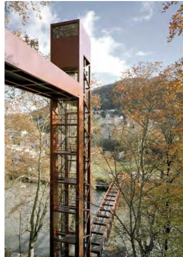
Gironella old town centre, Spain https://www.publicspace.org/works/-/project/249-new-lift-to-the-old-city-centre https://www.archdaily.com/776902/new-access-to-gironellas-historic-center
