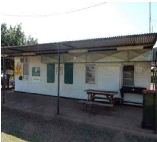
Kiosk and Office
