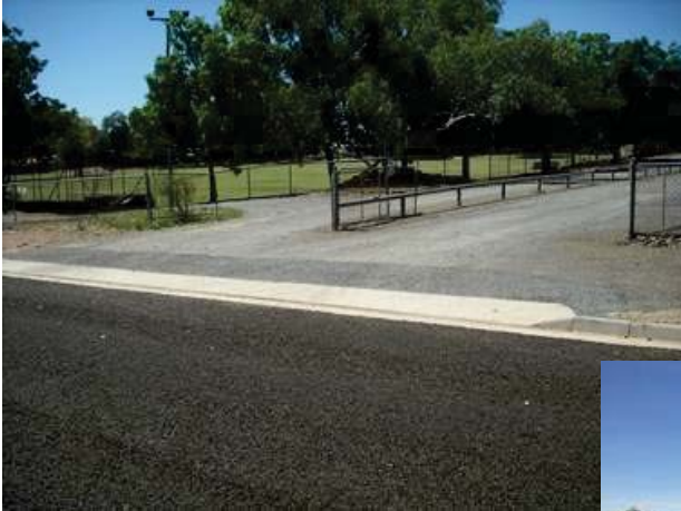
Pavement Rehabilitation Project
