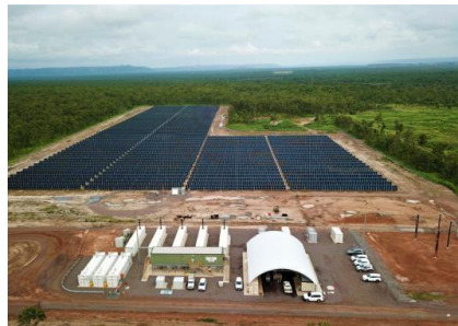
Figure 4-3: Representative solar + diesel + battery system
