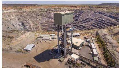
Figure 4-9: Representative QLD Copper Mine
