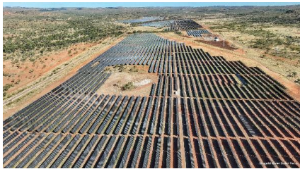
Figure 4-2: APA solar farm
