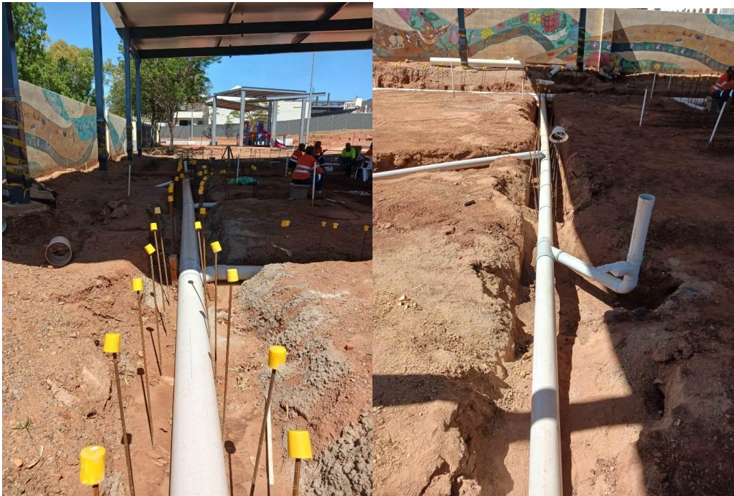
Figure 1 Drainage and plumbing installed ready for Concrete Pour on Tuesday
