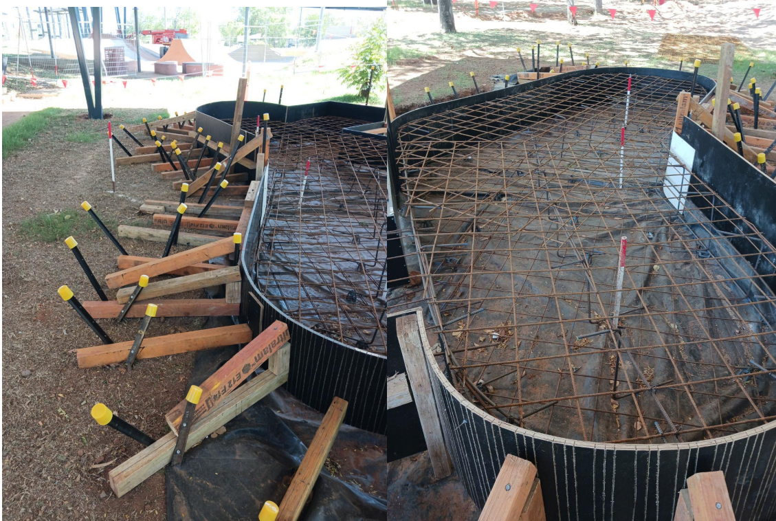
Figure 3Pre Pour Inspection for Main Stage
