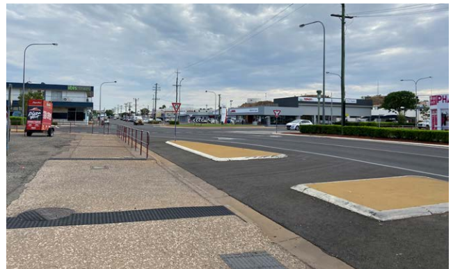
Figure 42. Site Photos of Streetscape and Carparking
