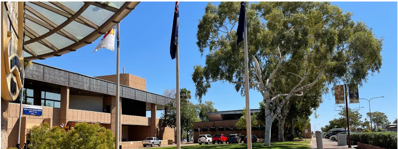
Image 16. Mount Isa civic centre and forecourt
