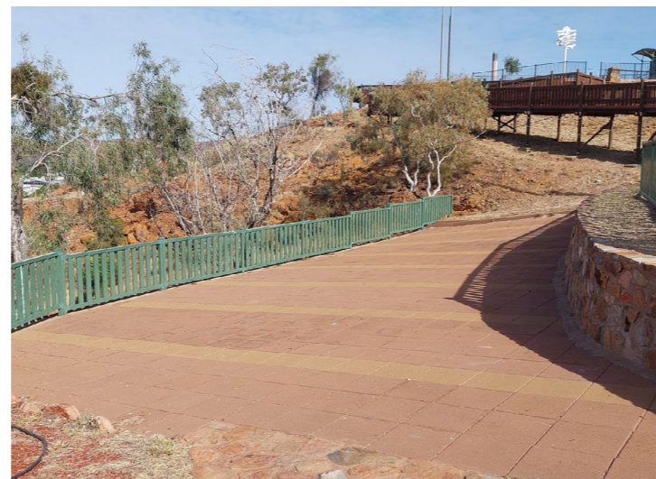
Unnecessary large paved and fenced area that appears to be disconnected from the lookout and it's purpose
