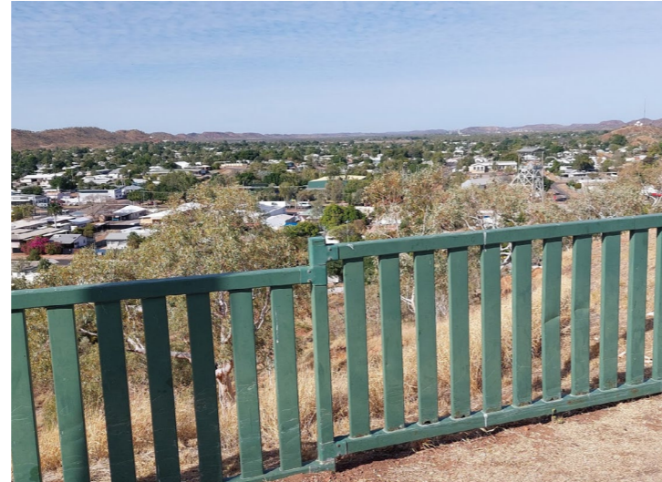
Excessive use of green fencing that is unsightly. The Fence is old and falling apart
