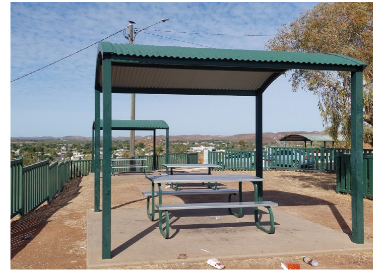
No Toilet facilities and drinking fountains. Structures are dated and unsightly.
