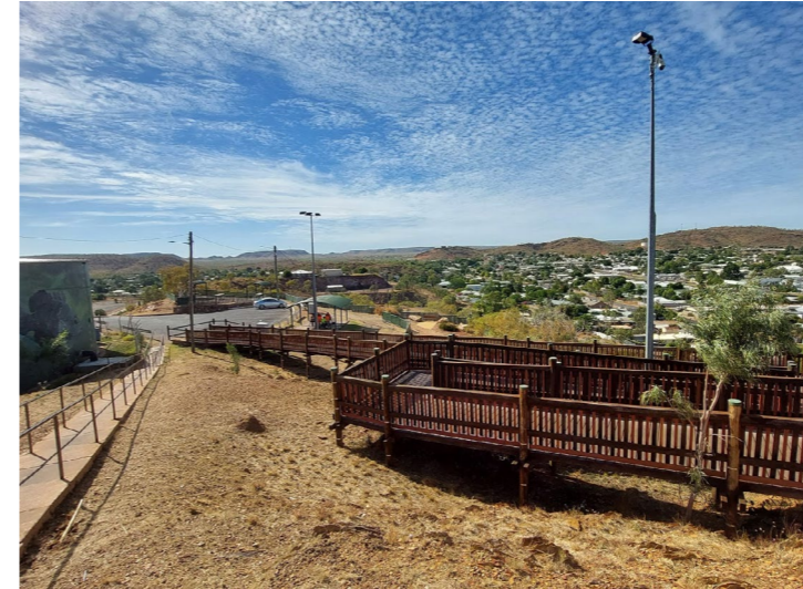
Two walkways up to the lookout is unnecessary. Boardwalk up to the lookout is old, unsightly, and falling apart. Pathway with metal fencing up to lookout is narrow unsightly.
