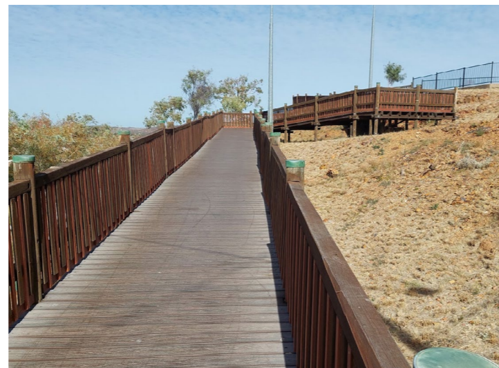
Ramp Accessible, however not up to current code.
